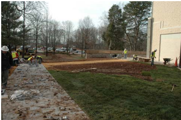
Terrace connection walkway and new sod
